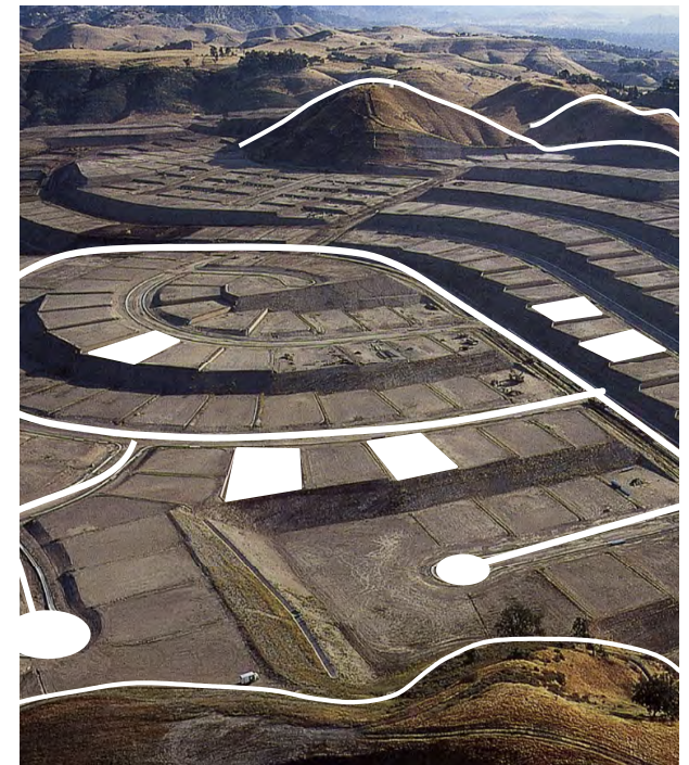
Site preparation for new hillside housing development
