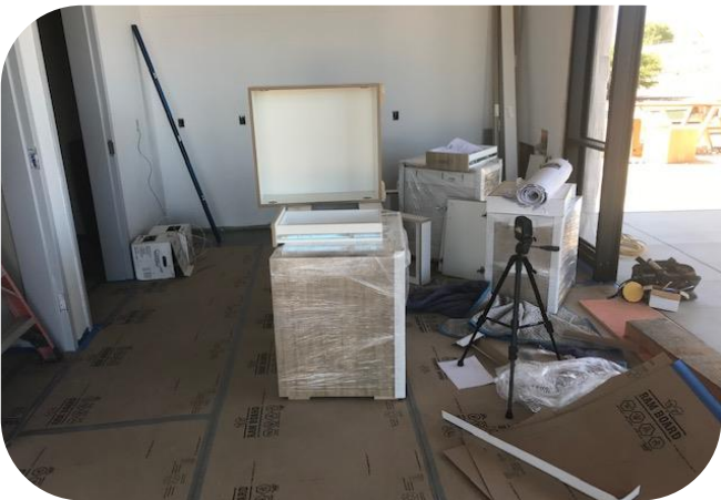
Casework on site.
