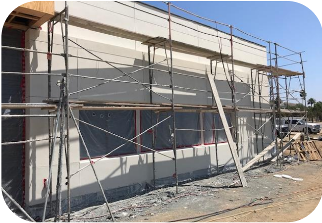
Plaster finish coat
