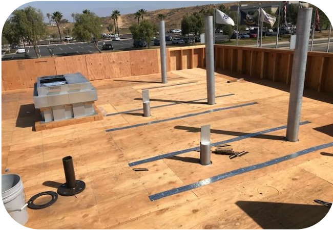
Bldg roof sheathing, strapping, curbs
