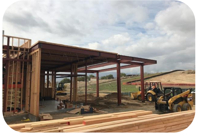
Finsh Grading at Patio
