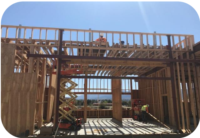
Roof joists/framing building
