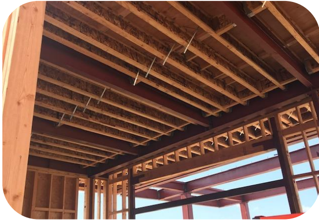
Lobby area joists/sheeting
