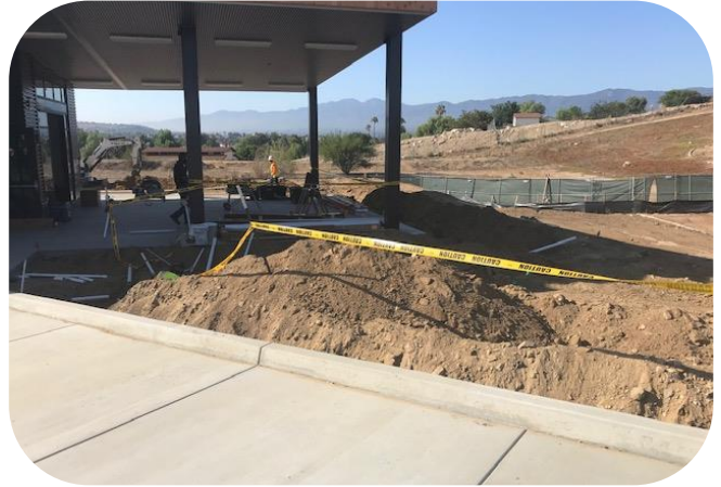
Irrigation Trenching
