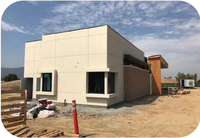
Plaster finish coat
