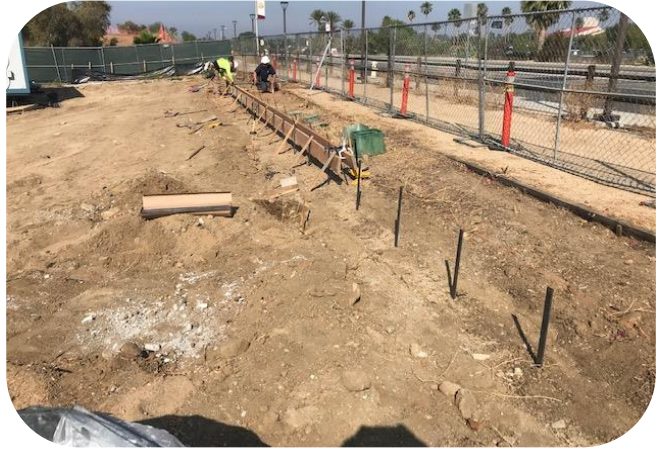
Curb formwork
