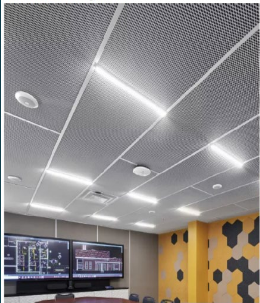
Metal Mesh Ceiling - Install
