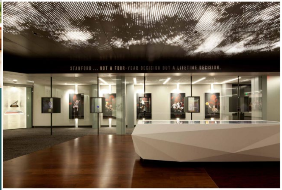
Perforated Metal Ceiling - Install
