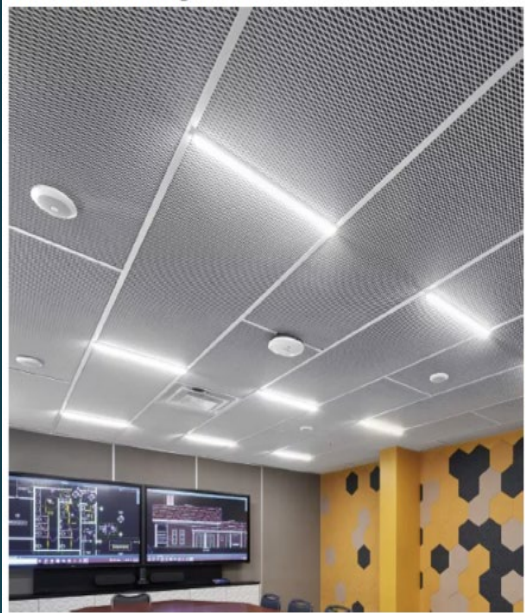
Metal Mesh Ceiling - Install
