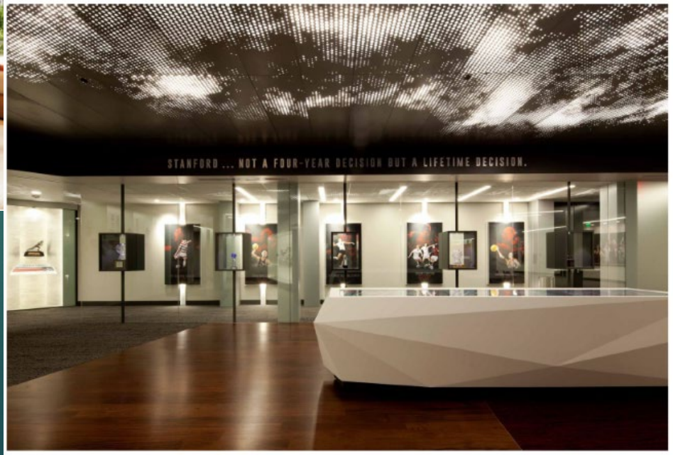
Perforated Metal Ceiling - Install
