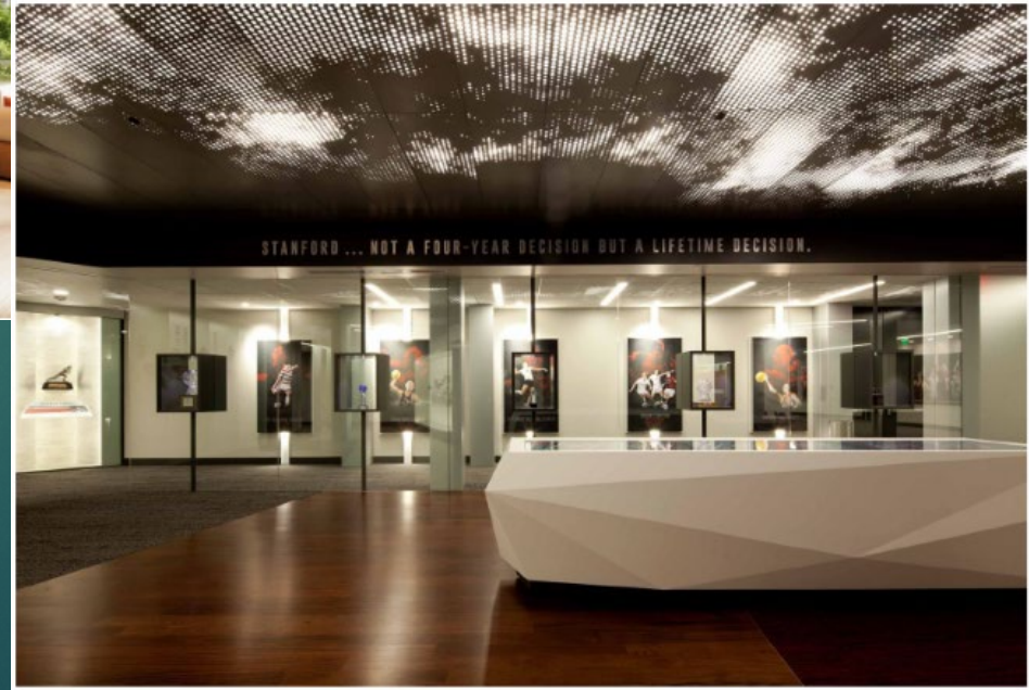
Perforated Metal Ceiling - Install
