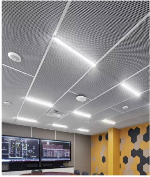
Metal Mesh Ceiling - Install
