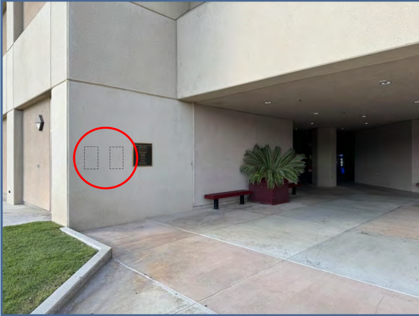
IT Building East Side
