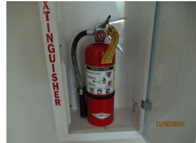
25. The employer shall be responsible for the inspection, maintenance and testing of all portable fire extinguishers in the workplace. Portable extinguishers shall be visually inspected monthly. CCR Title 8, 6151(e)(2)
