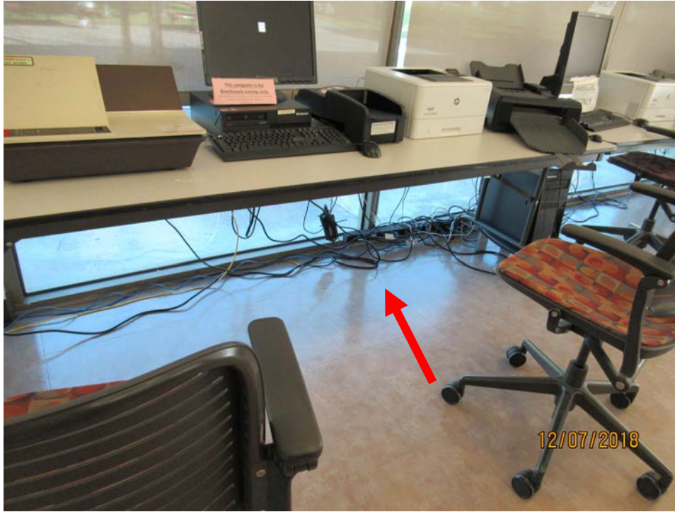
17. Bundle and constrain cords and cables under/around workstations. Eliminate use of piggy-backed power strips and extension cords. NFPA Section 11.1.4
