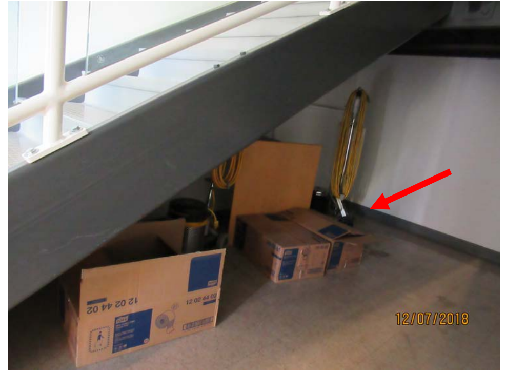
18. Remove storage under exit stairways. Uniform Fire Code (UFC) Section 1210.1
