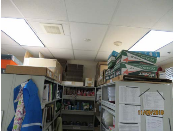
30. Maintain minimum 18-inch clearance between combustibles and ceiling. (with fire sprinklers) CCR Title 8, 6170(b)(10)
