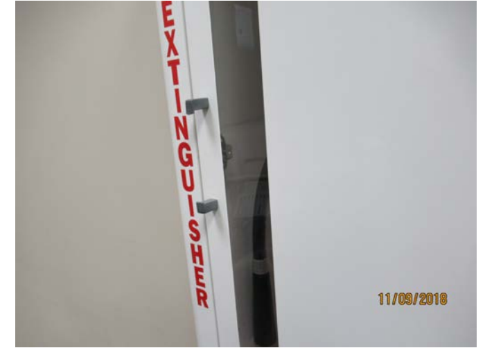
32. Replace broken handle on fire extinguisher cabinet.
