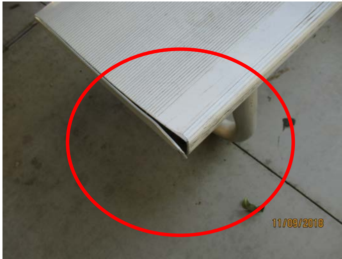
35. Repair damaged bench.
