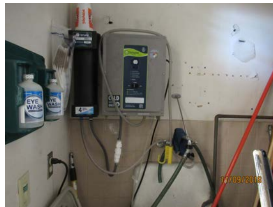
38. Provide emergency eyewash equipment. Eyewash must deliver 0.4 gallons of flushing fluid per minute for at least 15 minutes. ANSI Z358.1
