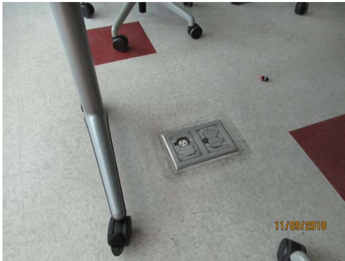
24. Replace missing cover on floor receptacle.
