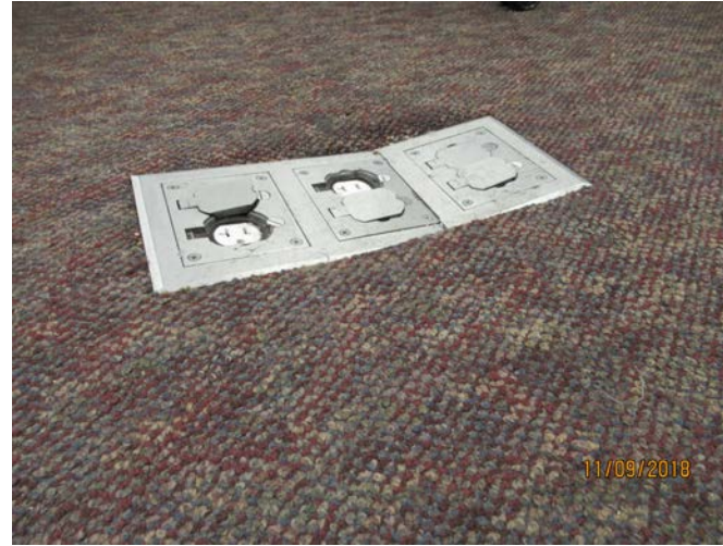
31. Replace missing cover on floor receptacle. Repair sloping floor.
