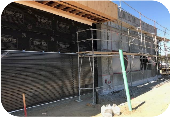
Metal Panels/ Plaster
