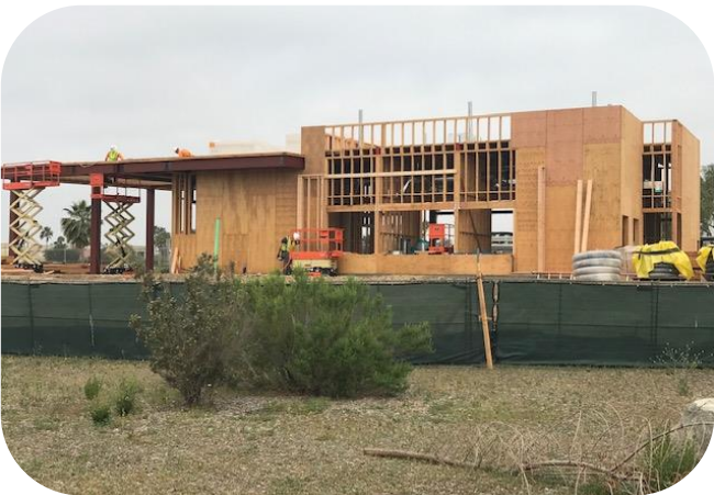
Roof Sheeting, Exterior Framing
