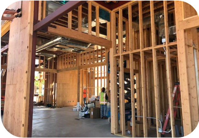
Interior electrical, ductwork rough in
