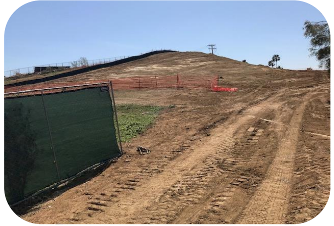
Borrow site finish grading
