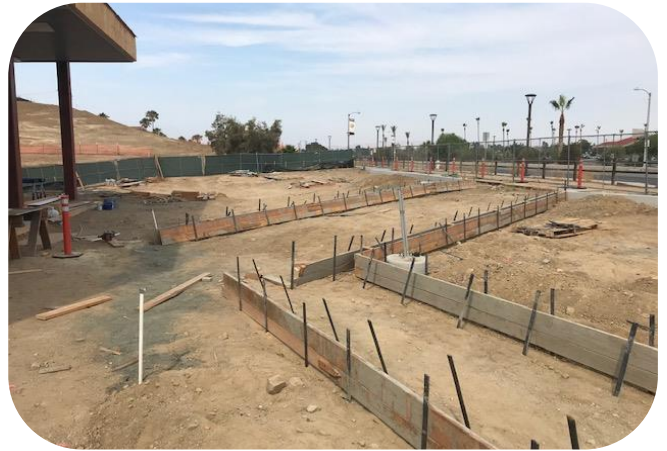
Curb Formwork
