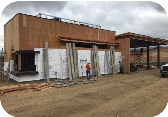
Waterproofing and scaffolding
