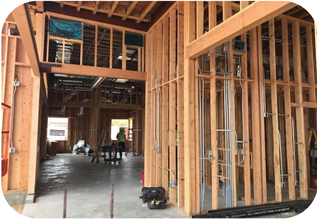
Electrical rough in
