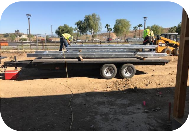
Rooftop Equipment Screen Frame
